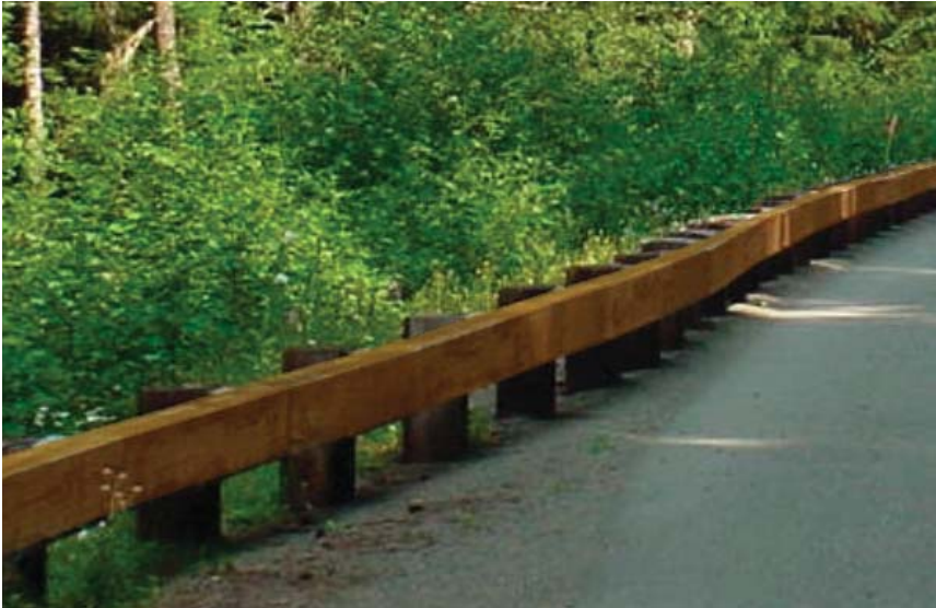
Figure 3.2-1 Guardrail: Steel-Backed Timber
