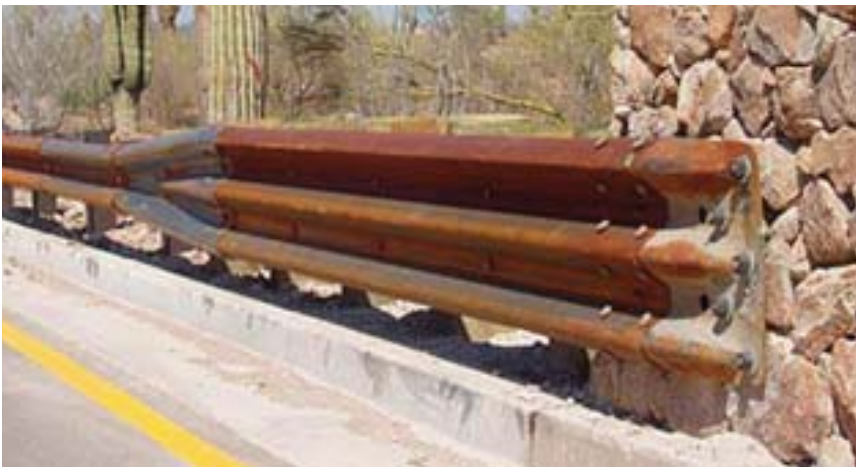
Figure 3.2-2 Guardrail: Weathering Steel
