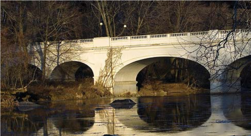
Figure 3.3-2 Bridge: Van Buren Street, Wilmington, DE
