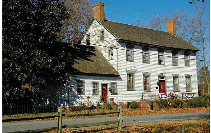
Cannon Hall, built in 1820, is the most prominent building on Woodland Village part of the byway.
