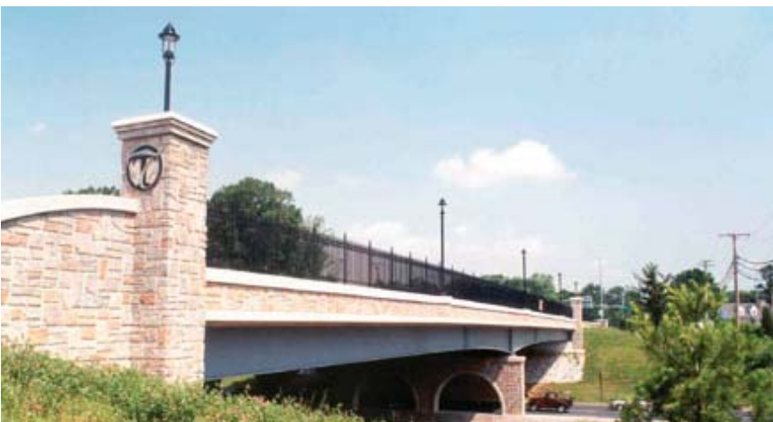
Figure 3.3-4 Bridge: Simulated Stone-faced Concrete, Dulaney Valley Road, MD
