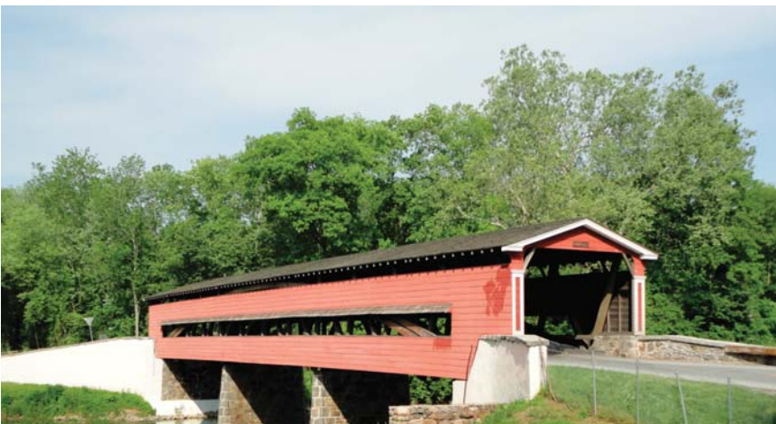
Figure 3.3-3 Bridge: Covered Smith's Bridge, New Castle County, DE
