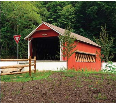
Figure 2.1-4 Functional Character - Wooddale Bridge, Red Clay Valley Scenic Byway, DE
