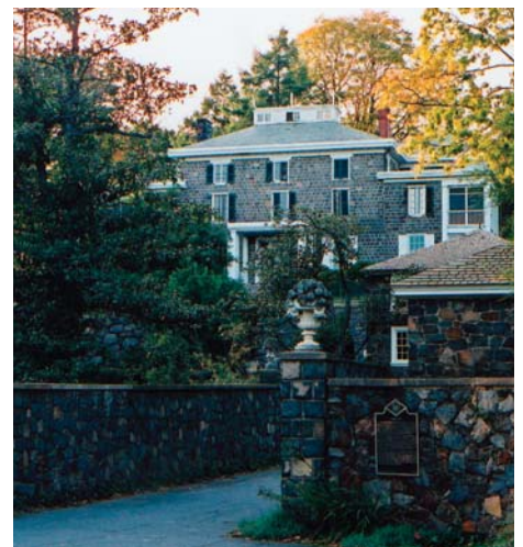
Figure 2.1-2 Historic Building - Gibraltar Mansion at Brandywine Valley National Scenic Byway, DE
